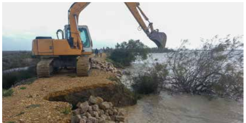
| Picture of an emergency intervention on a river levee during a storm event at Les Saintes-Maries-de-la-Mer
