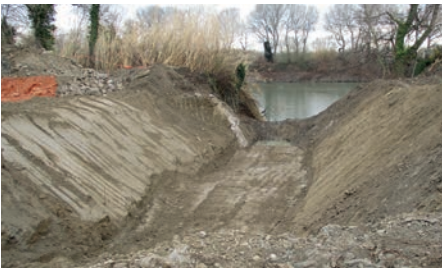
1 - Opening of excavations
