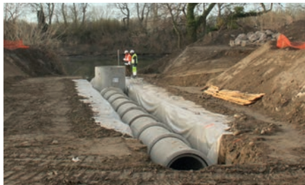
4 - Laying of the pipe
