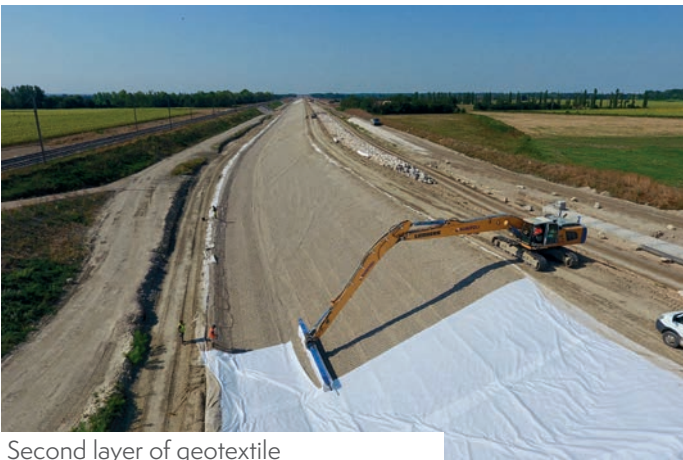
Second layer of geotextile
