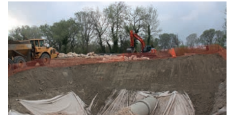
6 - Installation of the filter and downstream drain
