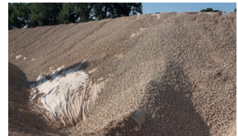
8 - Realisation of downstream drainage
