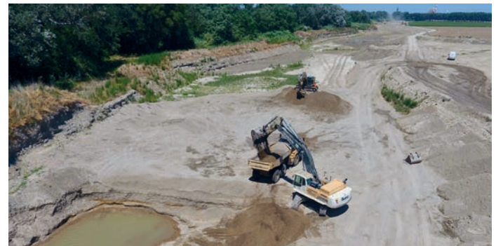
On-site material extraction and creation of a “lône”
