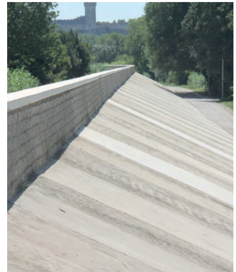
Montagnette levee, after work
