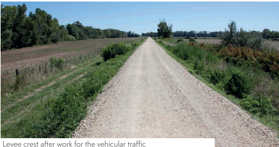
Levee crest after work for the vehicular traffic
