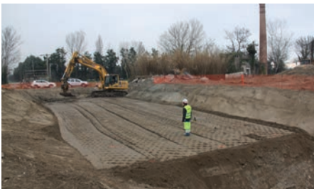
2 - Compaction of the foundation base
