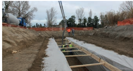
3 - Trenching and concreting of the excavation bottom
