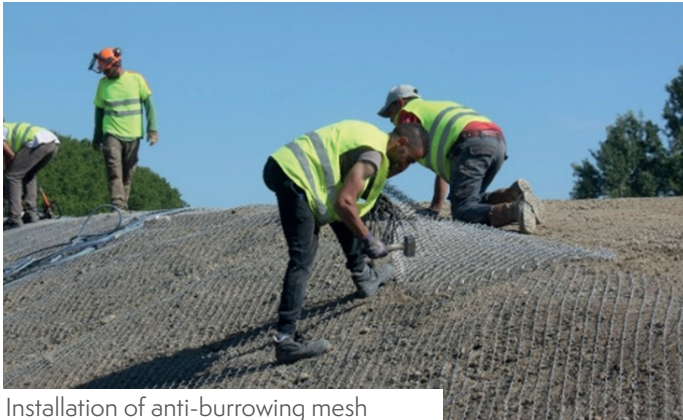
Installation of anti-burrowing mesh
