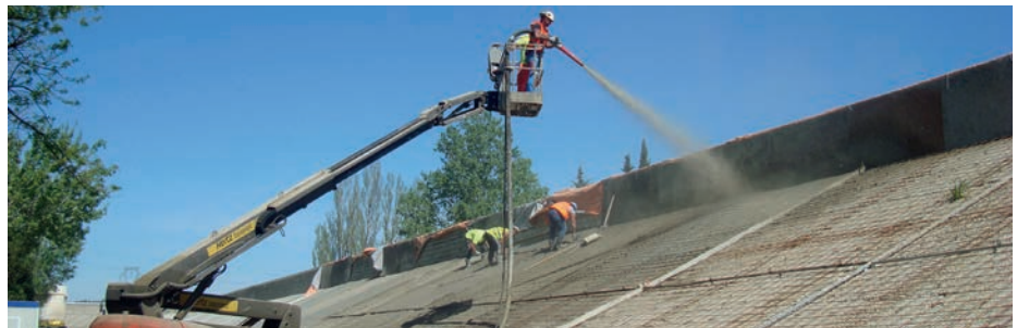
Montagnette levee, realisation of a waterproof siding in shotcrete
