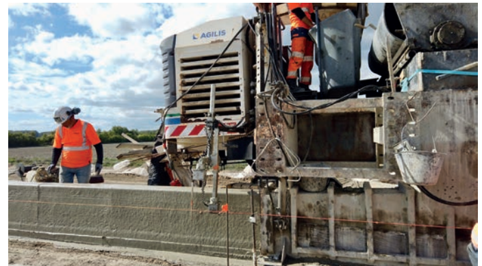
Concrete beam to determine the overflow level ...
