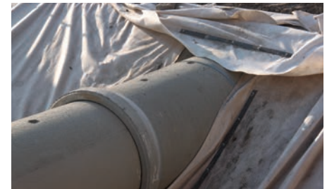
7 - Pipe filter link
