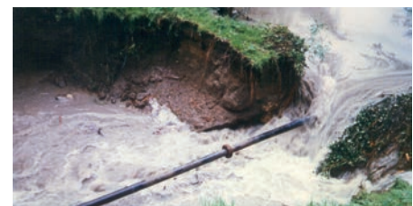
Breach caused by a crossing pipe
