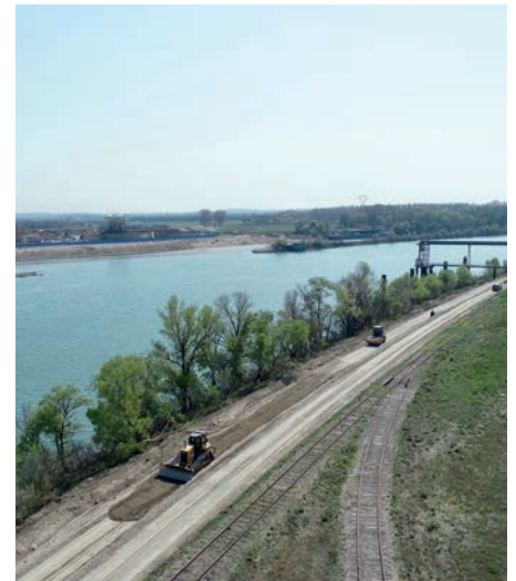
Works on the Industrial port site in Beaucaire
