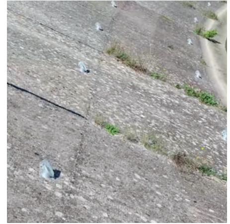
Drainage outlet, Boulbon spillway
