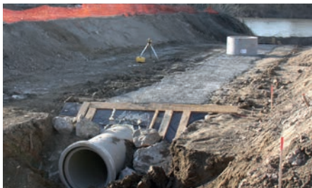
5 - Full excavation and coating concreting
