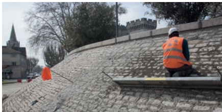
Montagnette levee, joining
