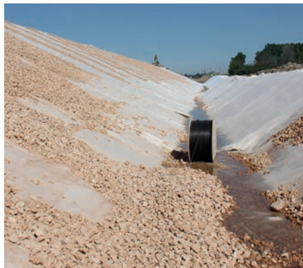
Laying of the optical fibre
