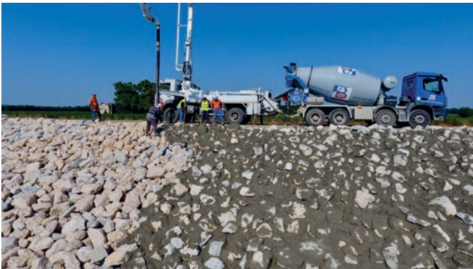
Concreting of riprap
