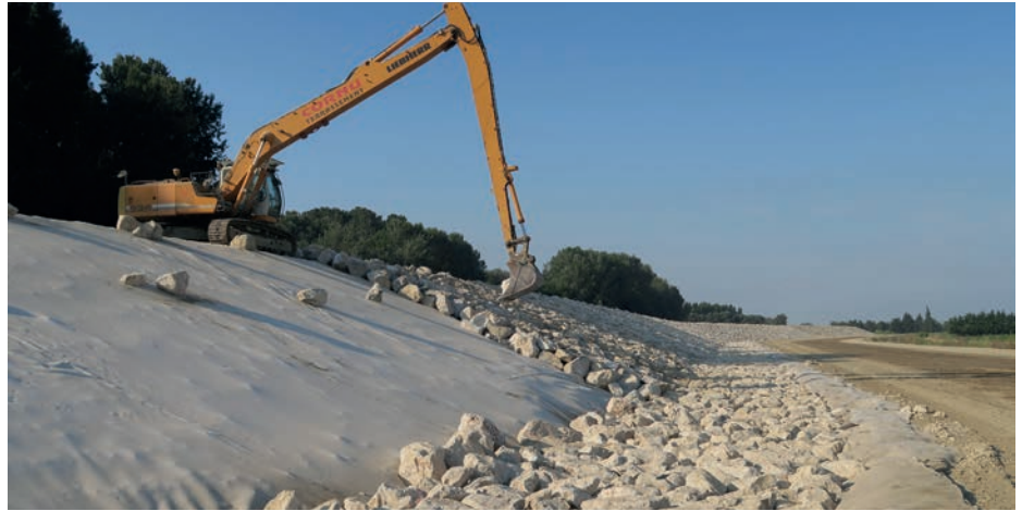
Laying of 200 to 400 kg riprap
