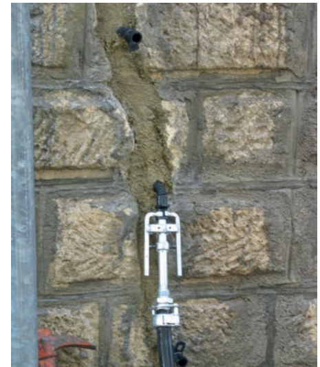
Banquette levee, clogged crack
