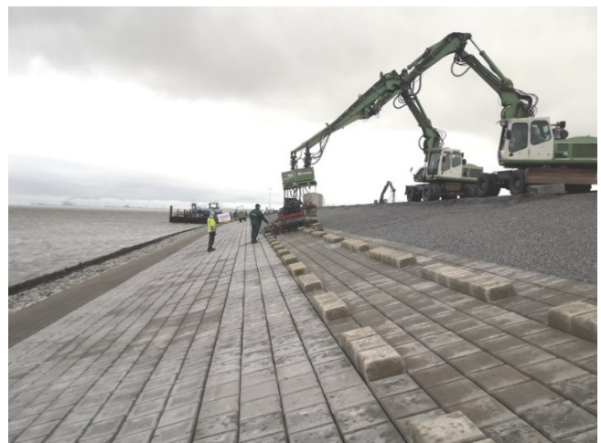
Figure 1 - Installation of the Verkalit® system
