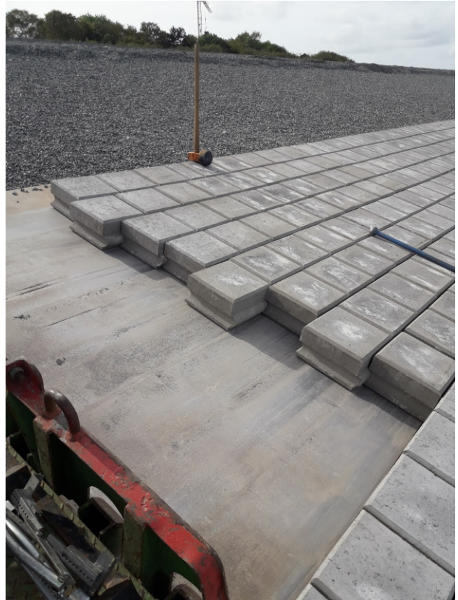
Figure 3 - Installation of the Verkalit® system
