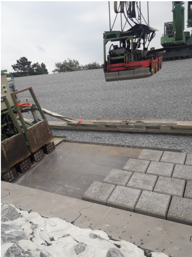
Figure 2 - Installation of the Verkalit® system
