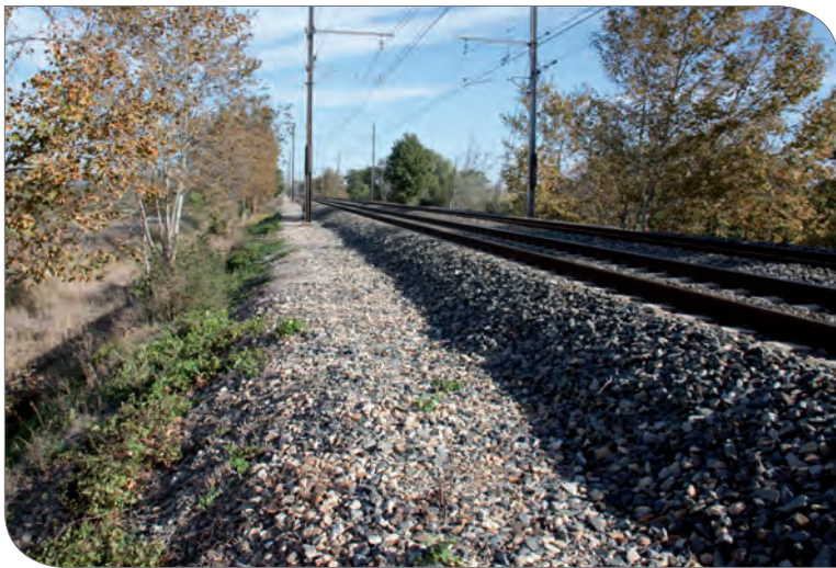
Remblai ferroviaire Tarascon/Arles (RFF)
